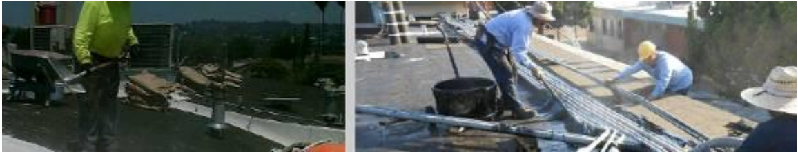
Workers replace roofs atop the District's schools.
